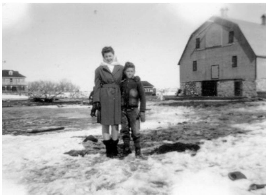
The photo above shows the reconfiguration of doorways as a result of the renovation to the horse barn. Also, just a bit of the henhouse can be seen on Clifford's left-hand side.
